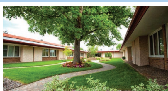
Courtyard renovation provided through the generosity of the M-Club.
